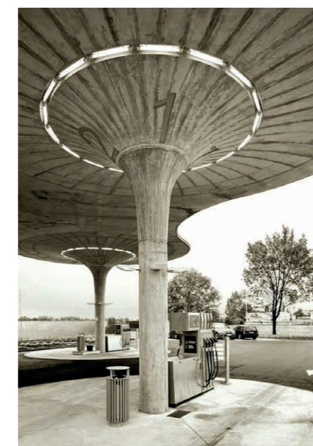
Petrol station GAS Matúškovo, Atelier SAD 2011
